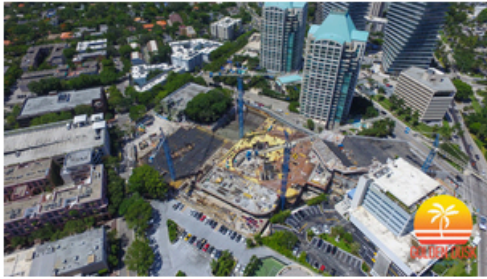
Construction on Park Grove
