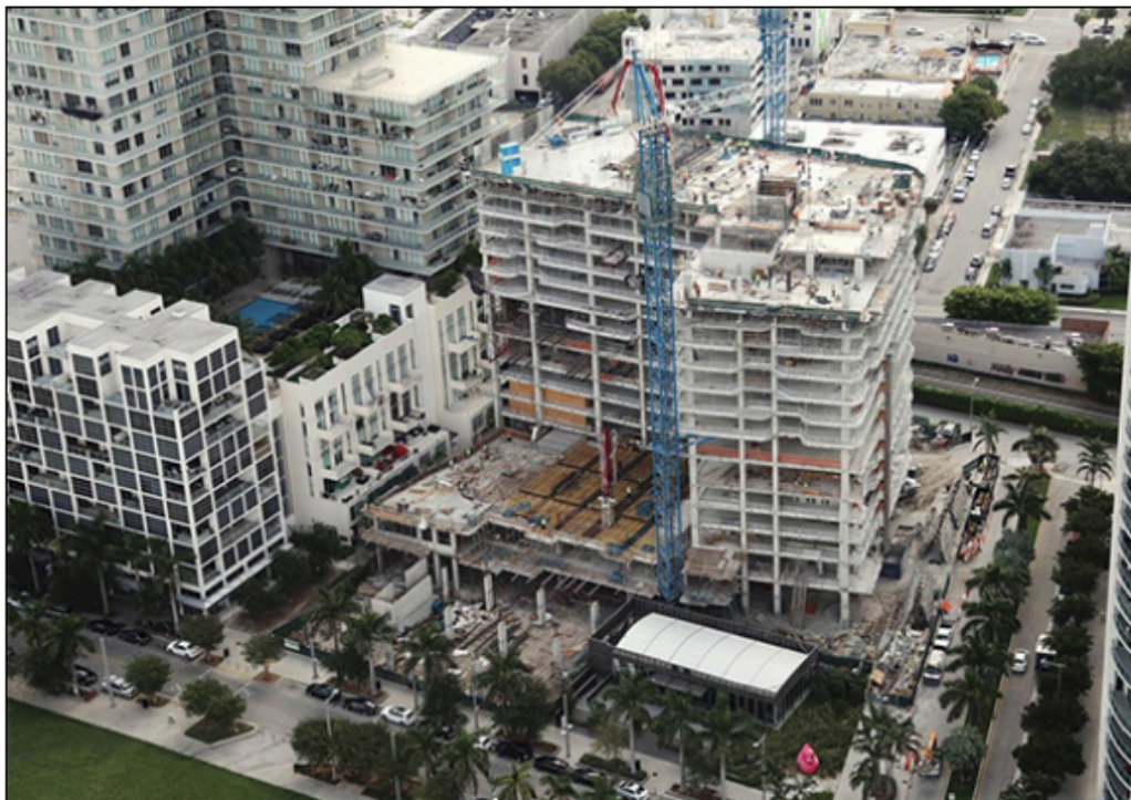
August photo of Hyde Midtown construction
