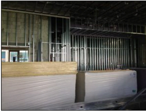
Interior of Michael Schwartz restaurant under construction
